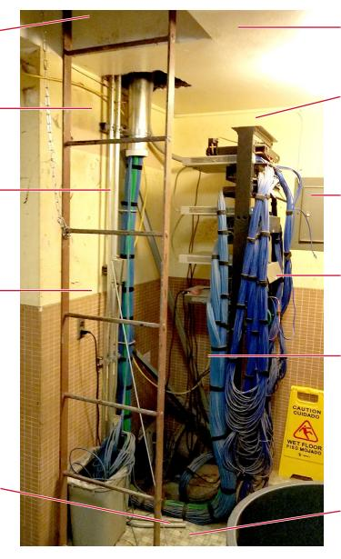
[12] Hard ceiling inhibits inspection and serviceability.
