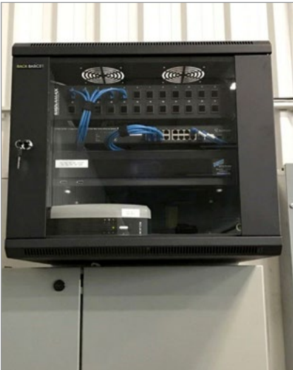
The wall-mounted IT equipment cabinet in the Computer Lab (MS Rm. 143) is in excellent condition.
