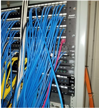
ES and MS horizontal cable management does not meet standards.
