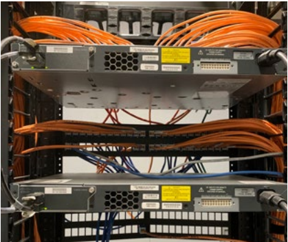
The rack in the MTR (MS Rm. 154) includes properly installed cable lengths and management.
