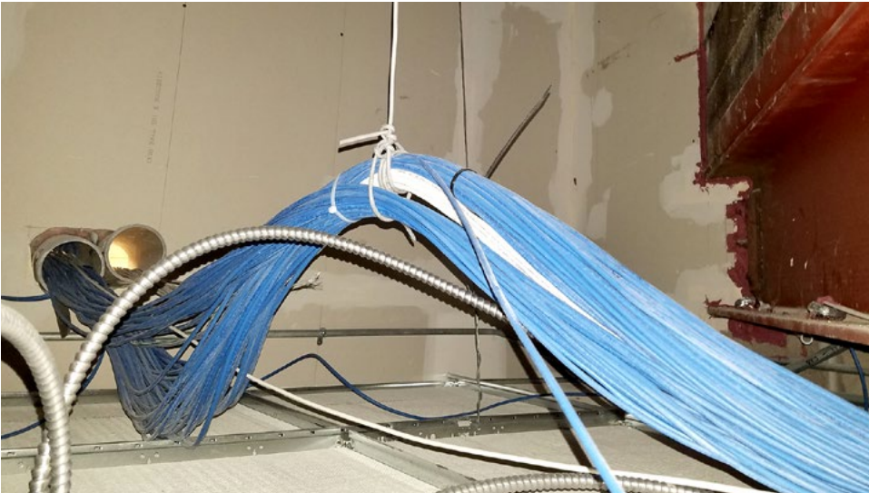
Example of improperly supported horizontal cable in the High School.
