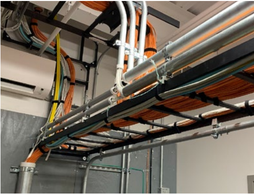
Ladder racking correctly installed and deployed in the Middle School MTR Rm. 154.
