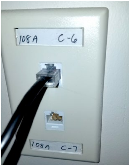
Typical ES and MS cabling with non-conforming labeling
