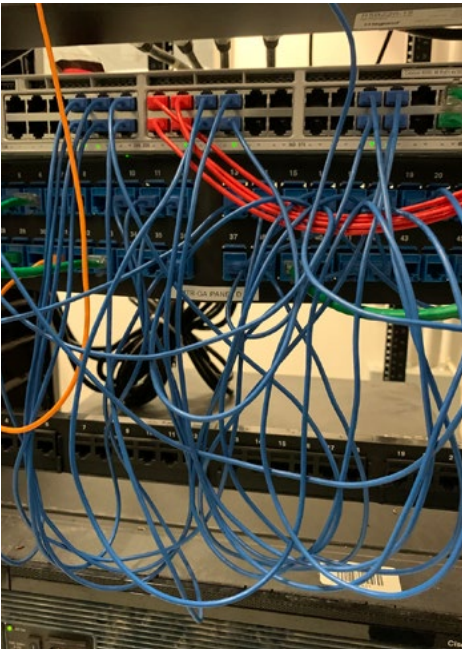
At left, one rack in the MTR (MS Rm. 154) show signs of “cable creep” in patch panels and server cables. At right, another rack in the same TR has correctly sized patch cords are neatly installed in machine-labeled ports.
