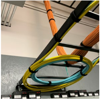
Ladder racking correctly installed and deployed in the Middle School MTR Rm. 154.
