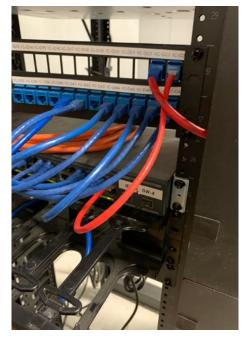
At left, one rack in the MTR (MS Rm. 154) show signs of "cable creep" in patch panels and server cables. At right, another rack in the same TR has correctly sized patch cords are neatly installed in machine-labeled ports.
